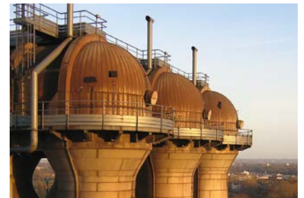
Blast furnace / stove dome
