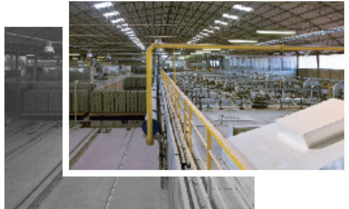
Pre-kiln and kiln roof with burners
