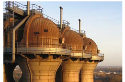
Blast furnace / stove dome
