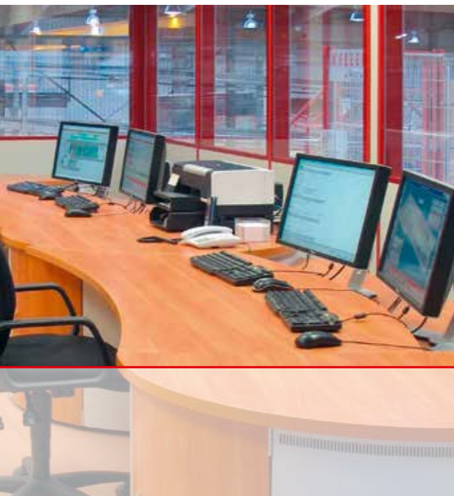
Air-conditioned switch room
