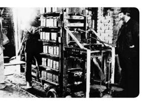
The finger car in the test phase. Instead of laths or pallets, they used boards that were placed by hand on the arms of the finger car. Then the bricks were placed and pushed on rails into the drying sheds.
